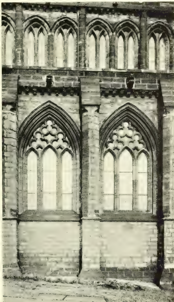
Bays in South Aisle of Nave (exterior)
